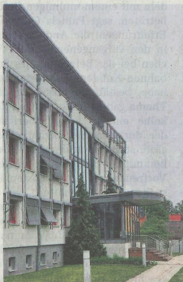
Das CCC in Harzgerode
